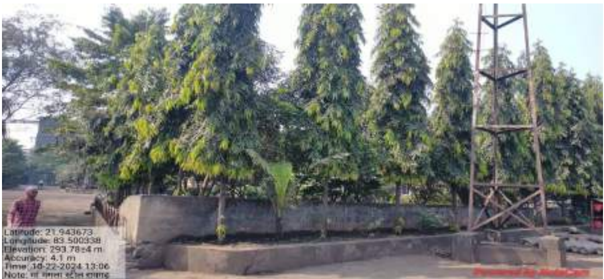
Coal washery in M/s Shiv Shakti Steel, Raigarh
