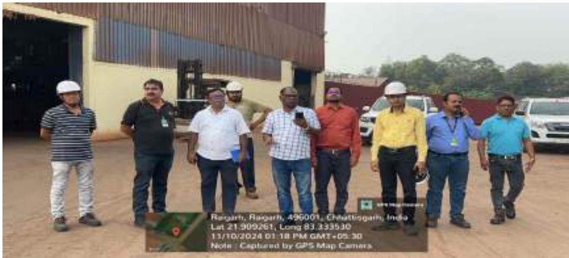
Fly ash brick manufacturing plant at M/s JSPL, Raigarh.
