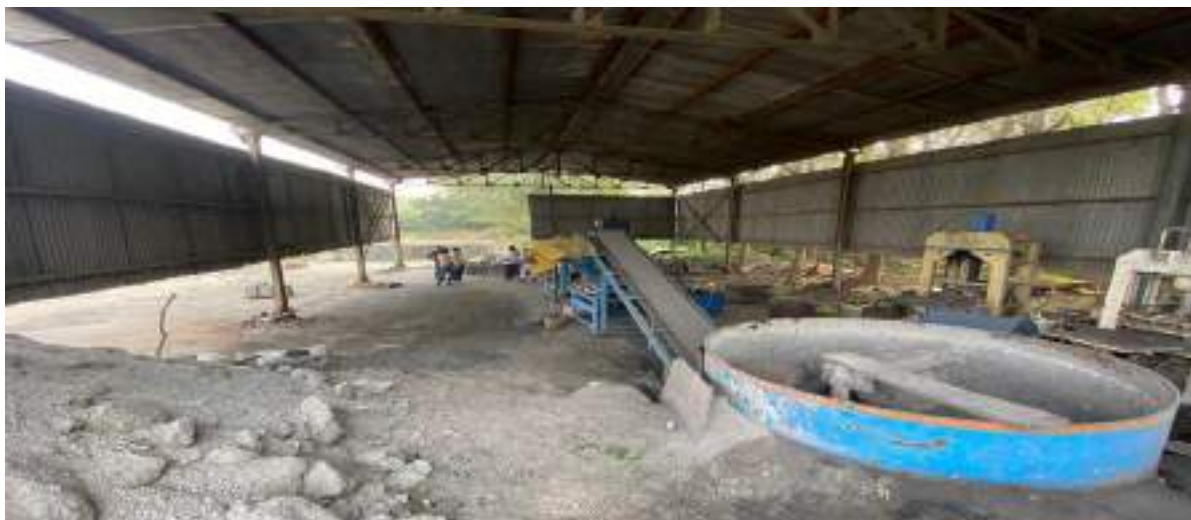
Fly ash utilisation in Brick plant of M/s Mahaveer Energy Ltd.
